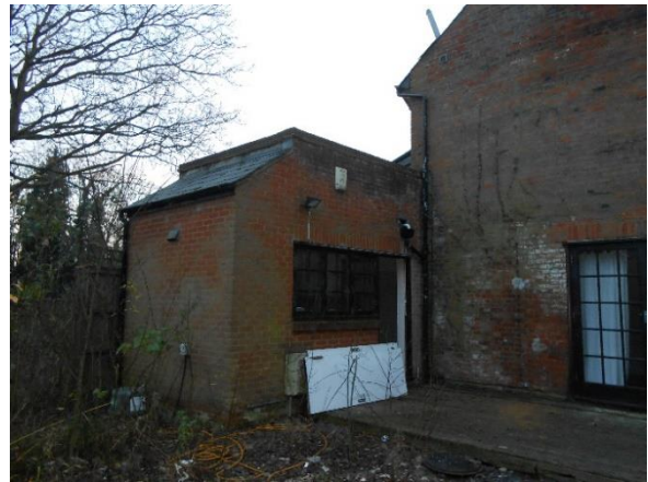
Figure 3 – Former extension to be demolished
